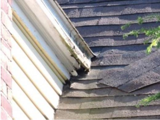
*The fascia and soffit boards of this cornice have rot due to moisture drawn from contact with the roofing. The resulting hole in the soffit on the underside of the cornice could serve as an entranceway for squirrels, causing additional damage to the building.*
