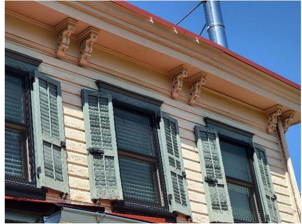
*Many types of wood elements are found throughout the VPA. This house has wooden eaves, brackets, siding, and shutters.*
