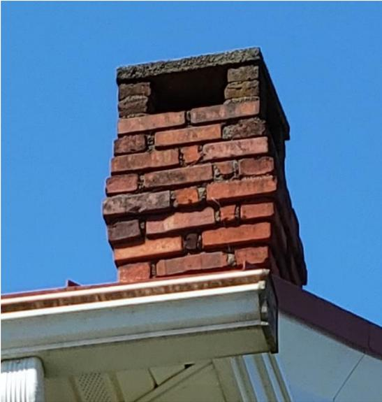
*A masonry plate was added to the top of this corbelled brick chimney to retard downdrafts and repel water. Although altering the historic appearance of the chimney, the design treatment is appropriate.*
