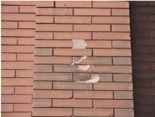
*The surfaces of these bricks have spalled, but the joints appear to be in good condition.*
