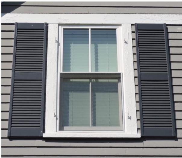
*In this example, despite the presence of authentic shutter hardware on the frame, shutters are mounted flat on the walls adjacent to the window, which could have been avoided.*
