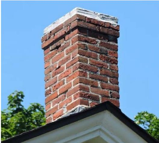
*The bricks in this chimney show their age – some are chipped and slightly spalled. They need not be repaired or replaced if they do not threaten the masonry as a whole.*
