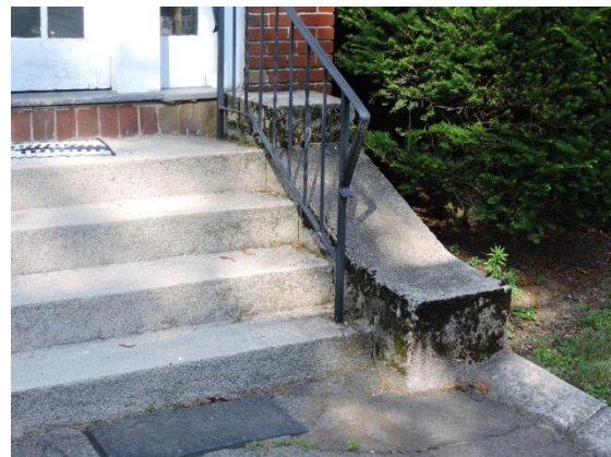
When installing metal handrails within the VPA, be mindful that their posts are susceptible to deterioration where they anchor into concrete or masonry. This can in-turn damage the surrounding concrete or masonry.
