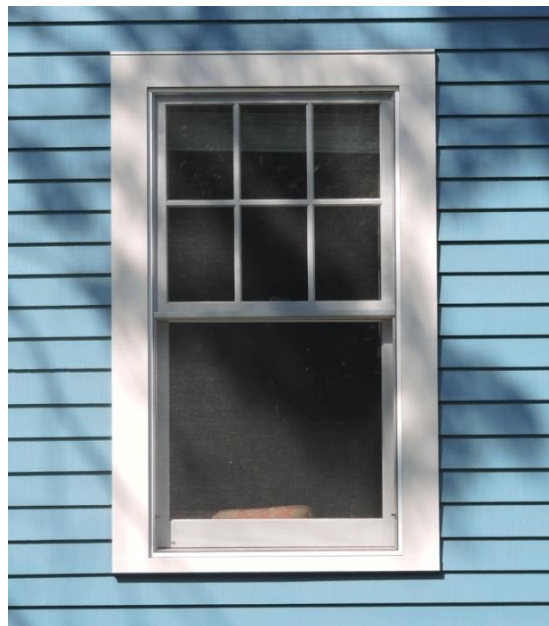
Replacement windows should match the full size of the historic window opening.
