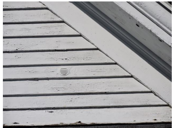
This siding shows indication of peeling paint. The small metal vent allows interior moisture to escape; retained moisture can eventually lead to interior rot and peeling paint, which can cause the wood siding to also rot.
