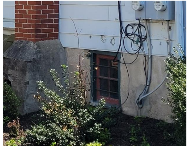
Stucco has been used as a protective coating over vulnerable masonry foundation walls
