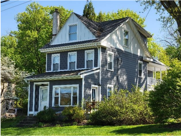
Cross-gabled roofs, as pictured, are not common on historic buildings within the VPA. Note the shed dormer at the rear of the building. (Joseph Grow House, 230 Byers Road).
