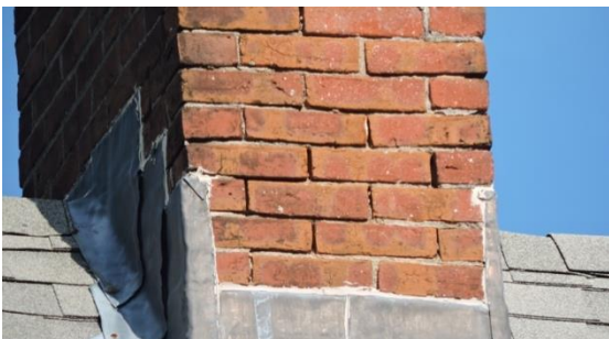
Open mortar joints may allow water to penetrate and deteriorate the brickwork.
