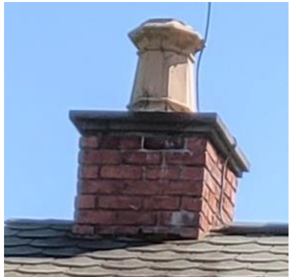
Common utilitarian chimney with original brick and terra cotta chimney pot.
