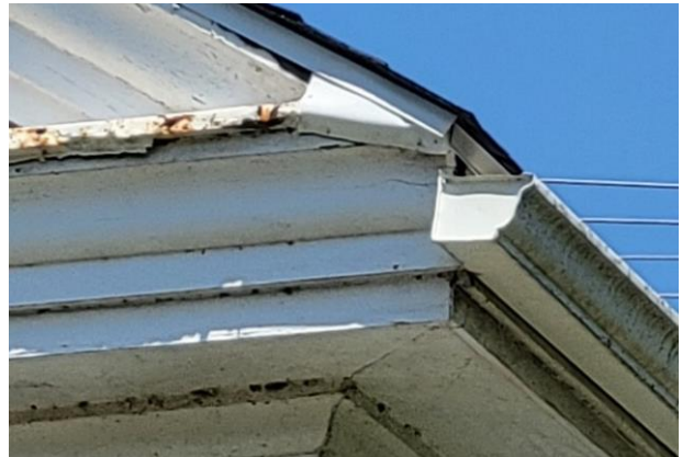
Contemporary K-style (molding shaped) gutter was installed on these buildings.
