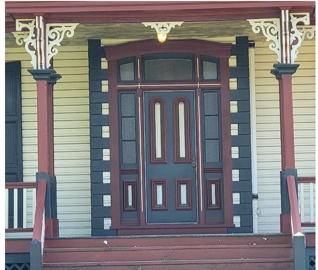
Historic wood doorway with solid paneled Italianate style door on the Todd House, displaying divided sidelights, transom, wood trim and wooden quoins.
