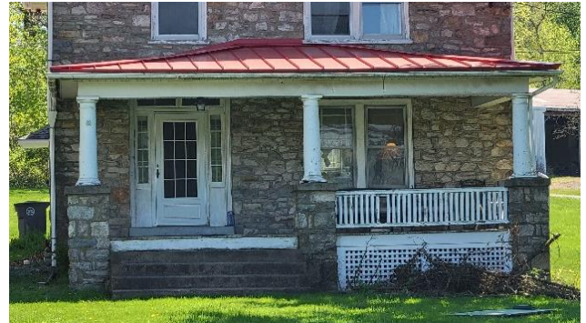
Wood porches are prominent features of many houses within the VPA. Exposed to the weather, their wood features require ongoing maintenance and occasional repair and replacement (Woodland House, 204 Byers Road, Byers Station Historic District).
