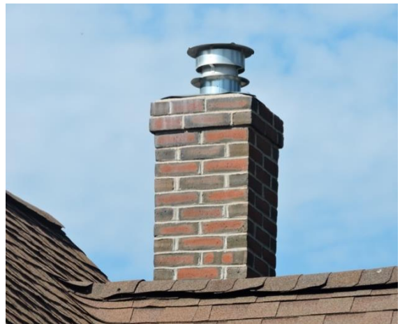
A variety of metal cap types have been installed on chimneys, not historic but acceptable for fire safety. This metal vent system is part of a rebuilt chimney with brick reasonably similar to the appearance of historic brick.
