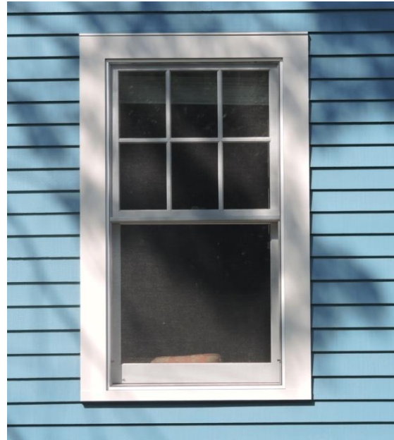
Replacement windows should match the full size of the historic window opening.
