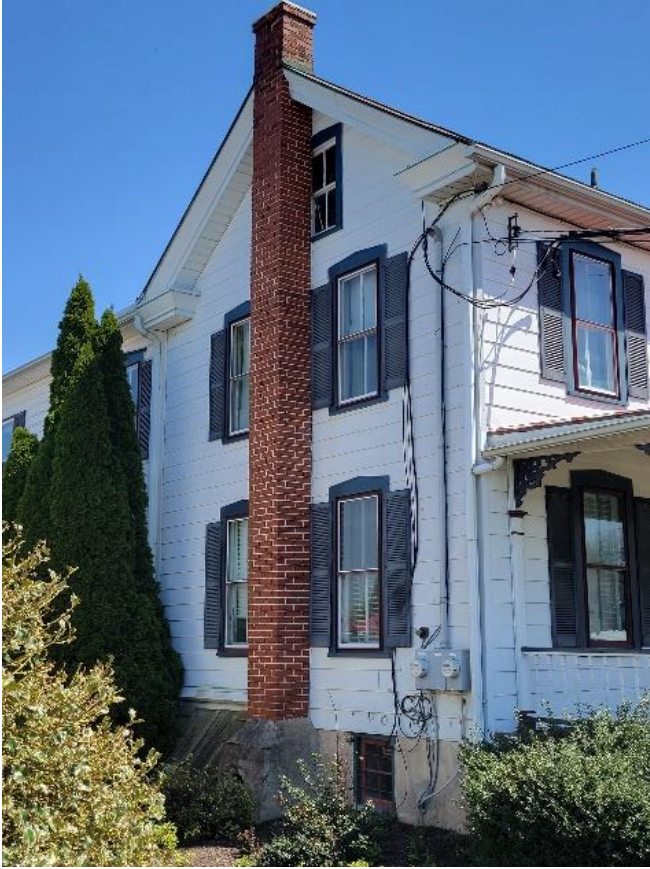
House in Eagle with a brick chimney (Isaac D. Frame House, 124 Pottstown Pike). The chimney was probably added in the twentieth century for an oil furnace.
