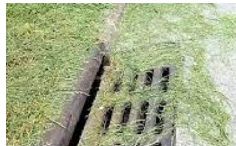
The grass ends up in the storm drains and causes them to backup or drain improperly. It can also lead to contamination in the waterways.
