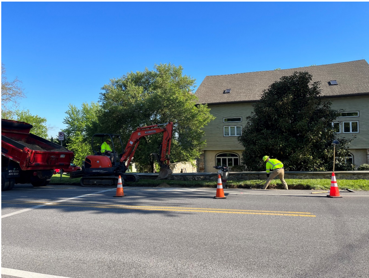
Park Road Project - May 2022
