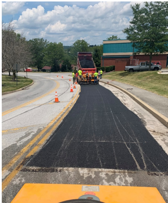
Base Repairs on Ticonderoga Road - August 2022
