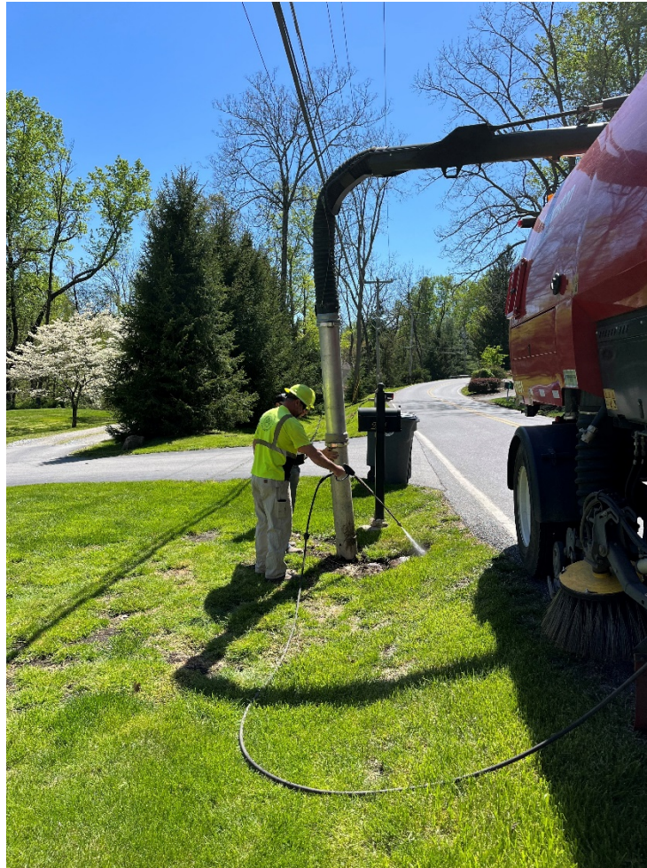
Vac Truck on Greenridge Road
