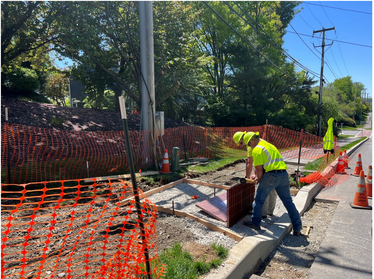
ADA Ramp installed on Park Road - May 2022
