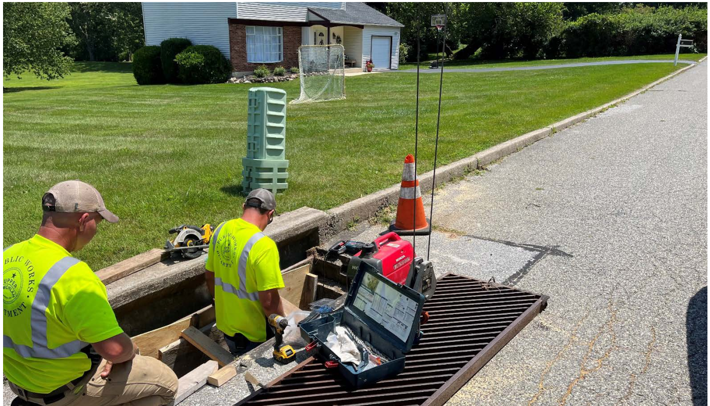
Waterview Road inlet repair - July 2022
