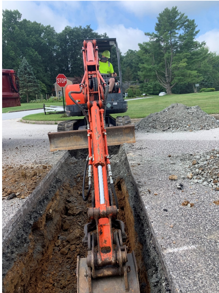
Pipe Replacement at the intersection of Fox Chase & Rabbit Run
